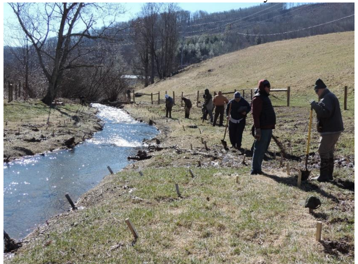
Photo Feb 2022 restoration day
