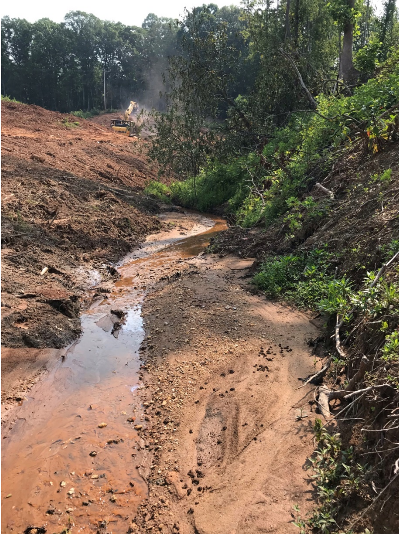
Photos 1 & 2: Extreme sediment deposits in stream channels causing complete destruction of channel geomorphology
